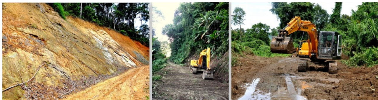
Figure 1. Showing the progressing road widening works in Maio-Vijoyanagar Road, Namdapha National Park.
